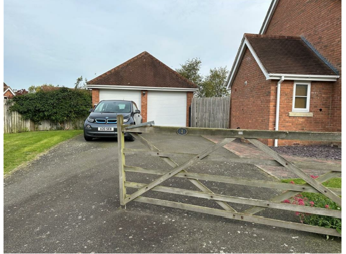
Double Garage 17'8" x 17'8" (5.38m x 5.38m)
